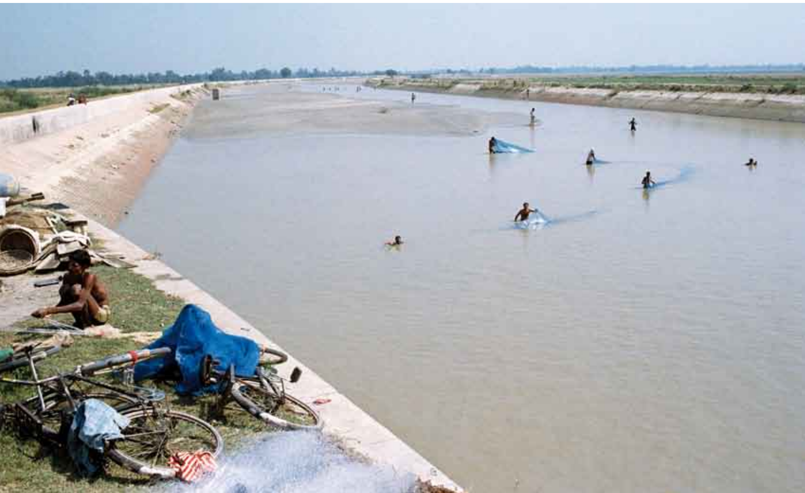
Siltation in Haidergarh Branch Head Canal, Uttar Pradesh. The silted canal now draws local fishermen.
